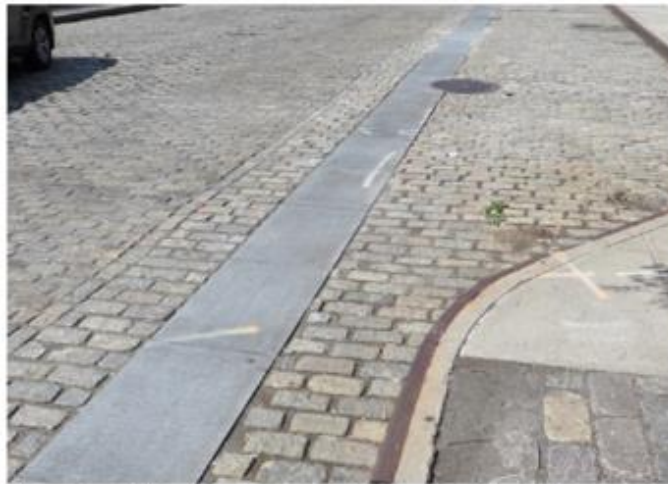
Figure 22: A bikeway on Varick Street in Tribeca, similar to the present proposed design for DUMBO's street reconstruction project
