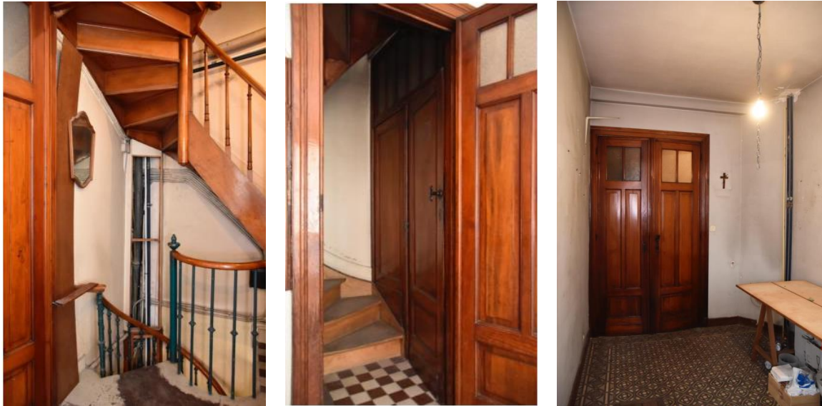
Portes palières © Archistory, 2019
