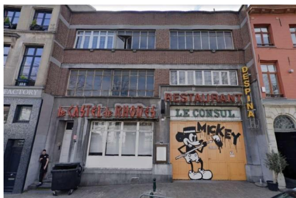
Gevel Baksteenkaai 38-40 © Google Streetview
