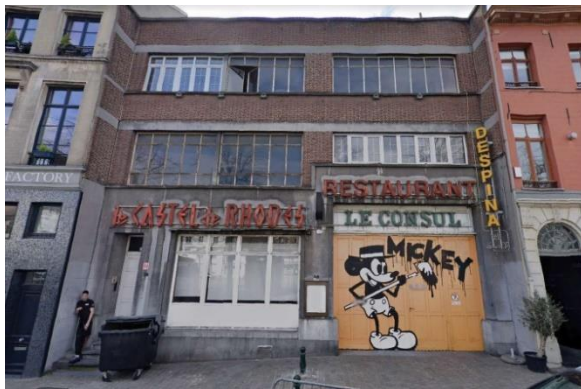
Gevel Baksteenkaai 38-40 © Google Streetview
