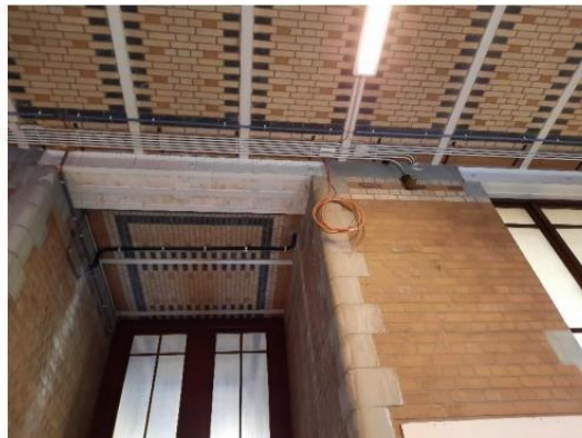
PHOTO J – Couloir C1.07
