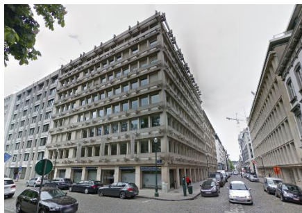
Situation existante (© Google Maps)
