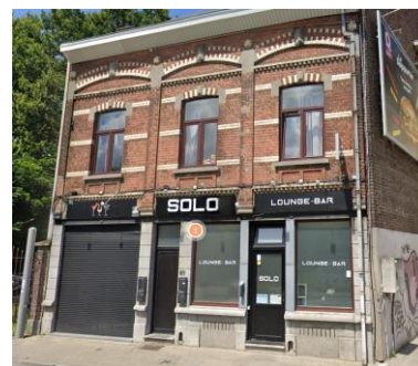
Situation existante – Photo Streetview
