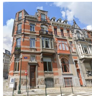
Façade Square Gutenberg. Photo existante 2024 ©Google Street View
