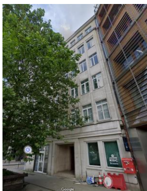
Situation existante ©Google Street view
